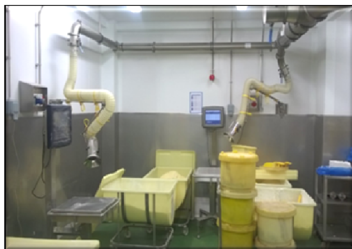
Example 9: Weighing stations with positional LEV captor hoods
