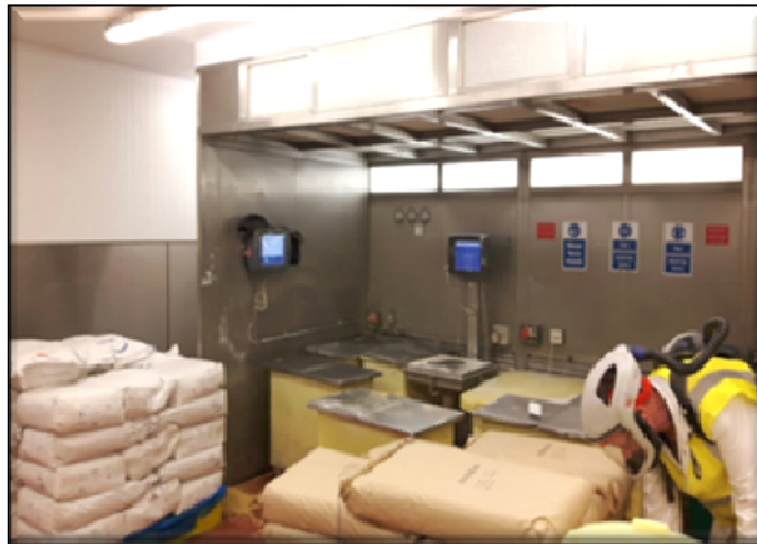
Example 2: Weighing stations in LEV booth
